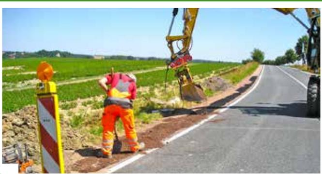
**3** COVER UP TO THE EDGE OF GEOROAD WITH FINE-GRAINED. IT IS POSSIBLE TO COVER THE SURFACE WITH GRASS, TOO.
