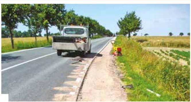
**1** APPLY A SUPPORTING LAYER WHICH CAN WITHSTAND TO THE STRESS OF THE TRANSITING VEHICLES
