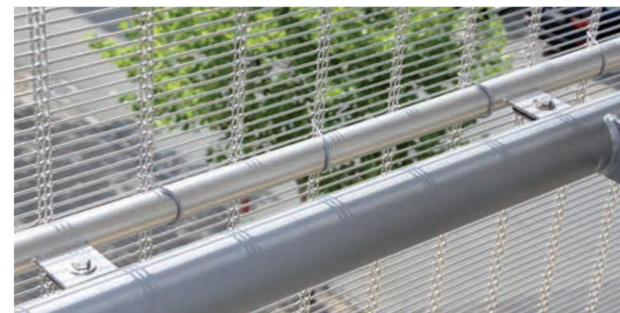
Intermediate mounting: round tube and wire connectors.
