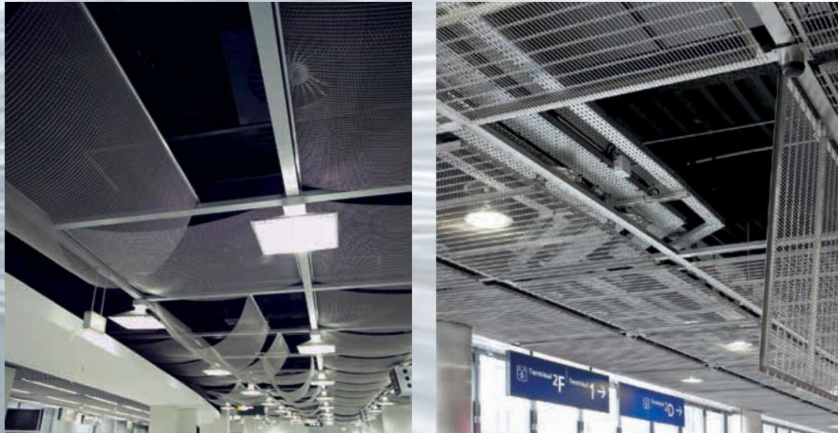
Adjustable mounting system for ceilings with sag.
