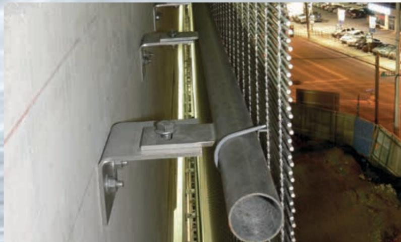
Intermediate mounting: round tube and wire connectors.
